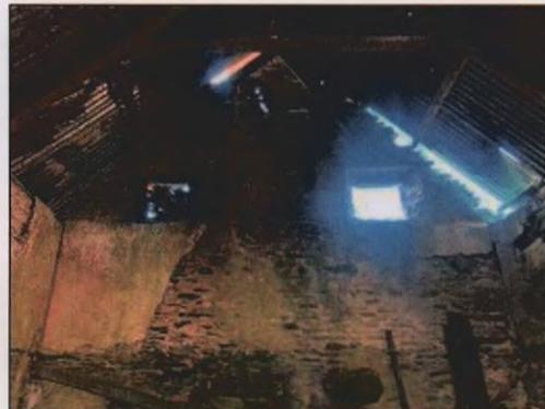
Plate 4-2 The interior of the structure (north-east wall), showing the open window, gaps in stonework and gaps under the roof.
